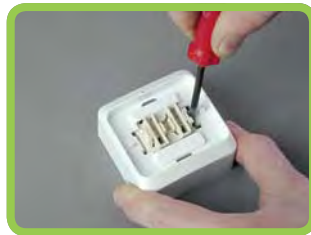
P116742 Lever the cover snaps on both sides of the insert, pushing the screwdriver handle towards the centre of the switch, and remove the cover.
