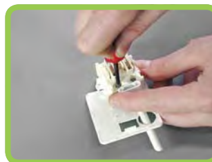
P116745 Connect wires to the terminals according to the markings on the back of the insert.
