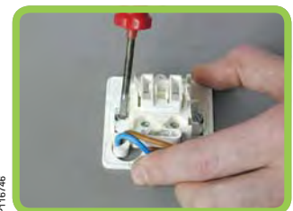
P116746 Snap the insert onto the backplate and fix the insert to the wall with screws. Distance between screws: 38 mm.
