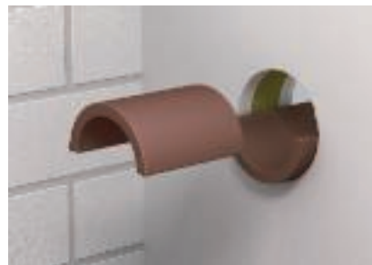
Torukesta paigaldamine kergesse vaheseina
