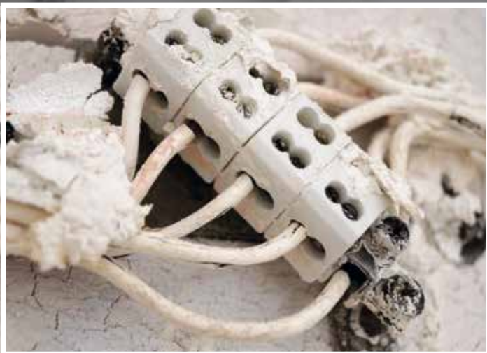
Even though the plastic enclosure has melted, the current is still flowing.
