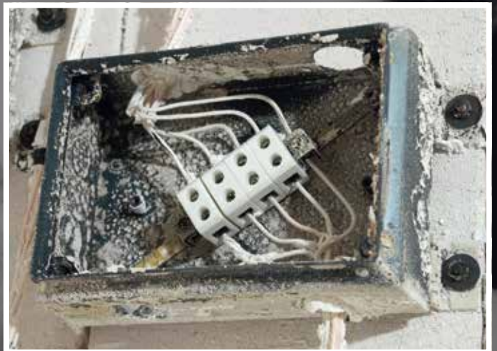
Metal enclosures and ceramic terminals remain in good condition.
