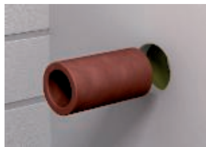
Torukesta paigaldamine kergesse vaheseina
