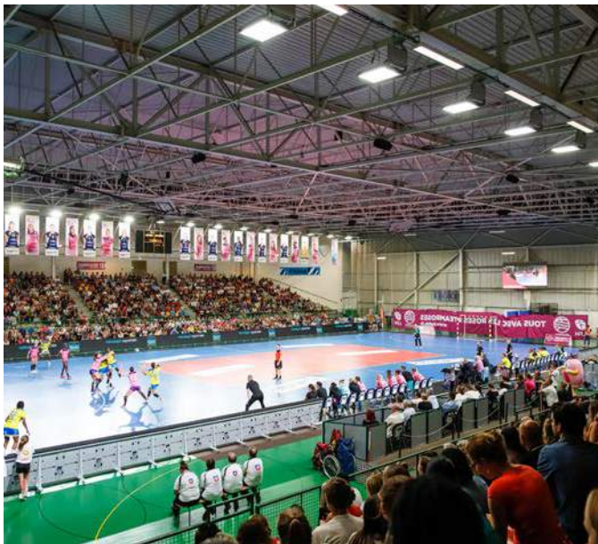
Mangin beaulieu sports complex - Nantes - France
