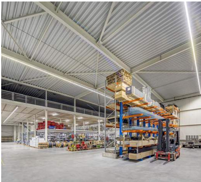
New building electrical wholesaler robri - Wekerom - Netherlands
