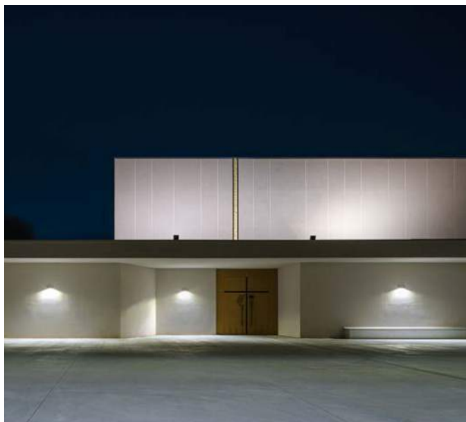
Parish complex - Varignano - Viareggio - Italy
