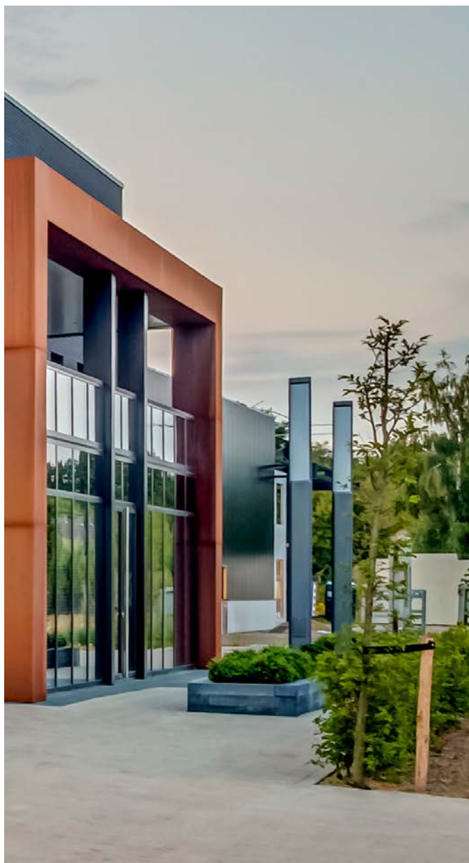
New building electrical wholesaler Robri - Wekerom - Netherlands
