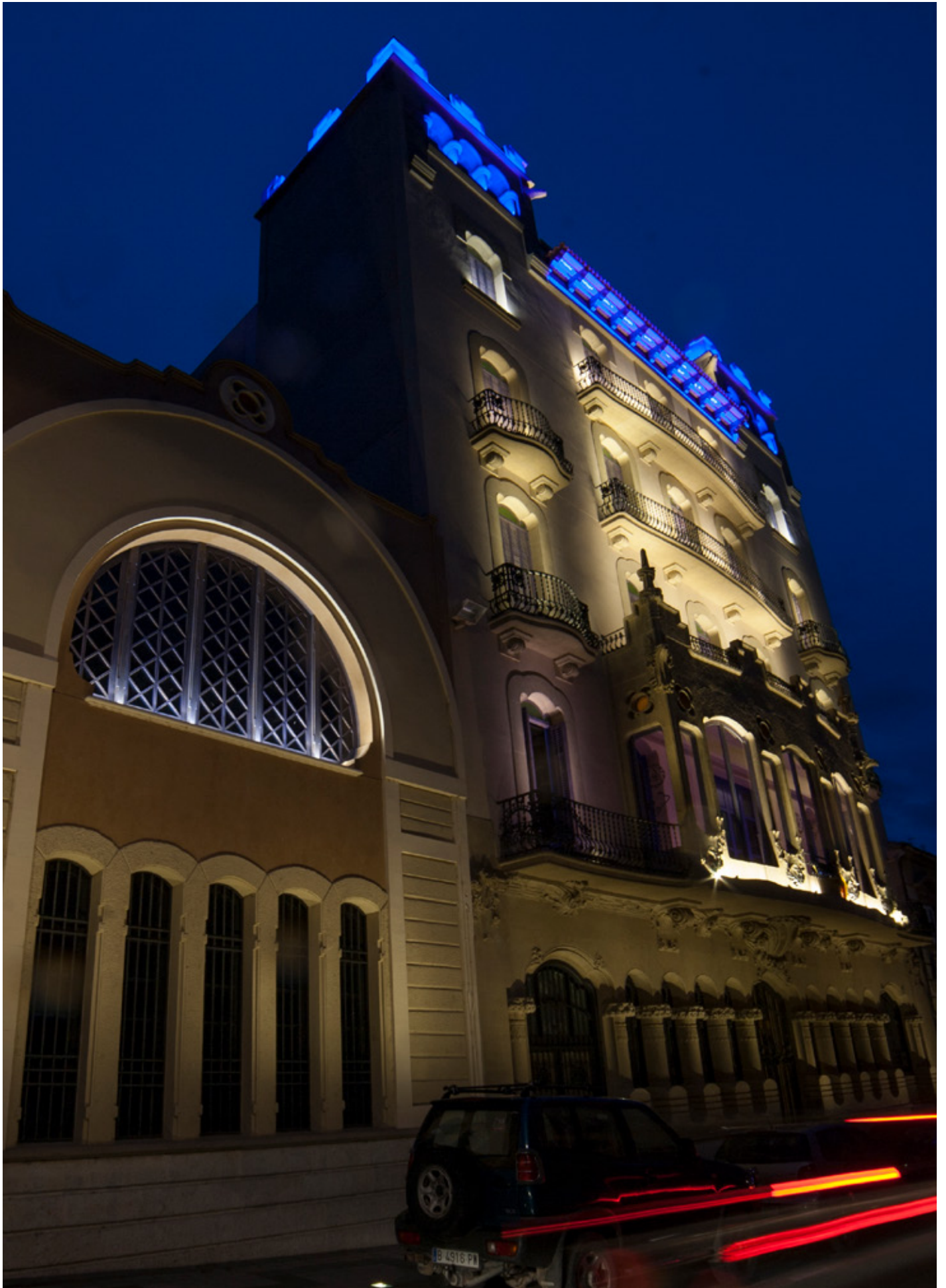
Casa Bau | Tortosa | Spain
